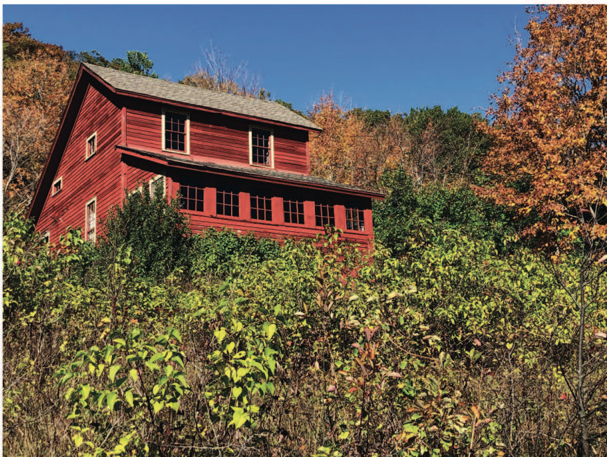
Long-abandoned mine shafts, crumbling industrial structures, workers' homes and gravestones of mining accident victims are reminders of the Keweenaw's copper glory days. (Photo by Kath Usitalo)
